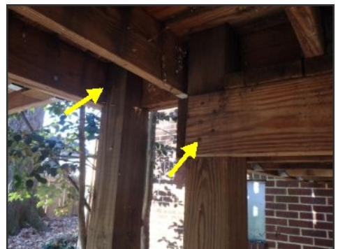
beams not bolted to support posts--example
