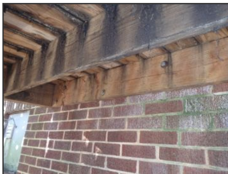
decks should not be bolted through brick
