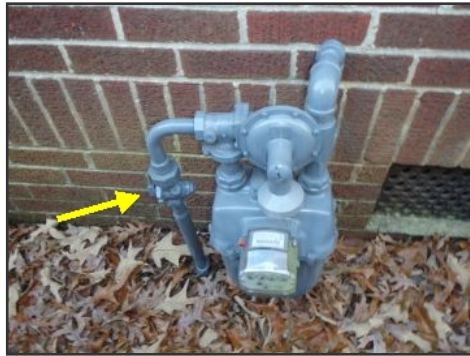
main gas valve
