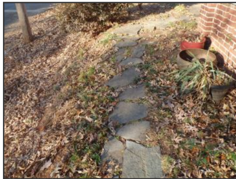
walkway on side D
