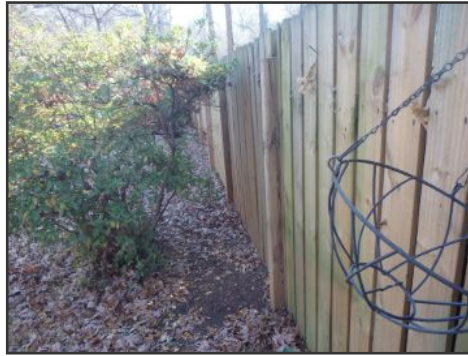
general image of fence
