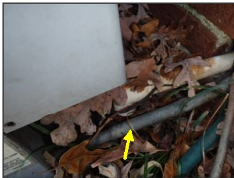
missing insulation
