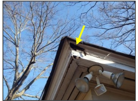
wood deterioration at side A
