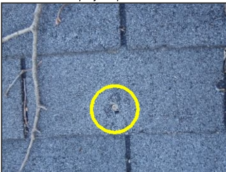
example damaged area
