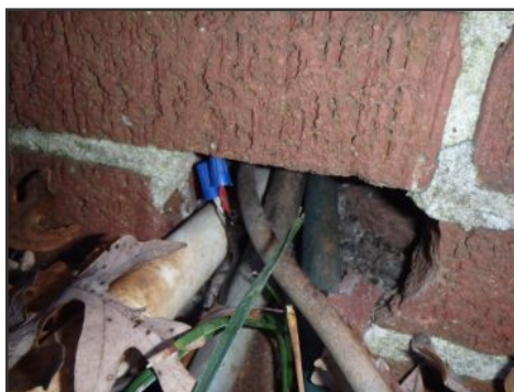
gap could allow rodent entry--side C
