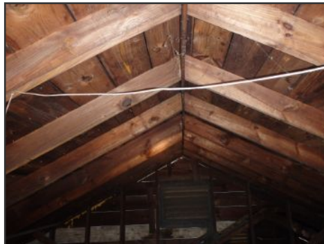
no collar ties are installed
