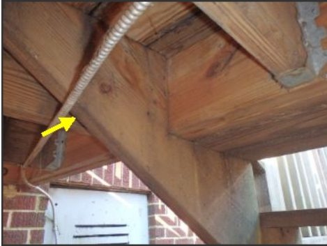
deficient attachment of stair stringers
