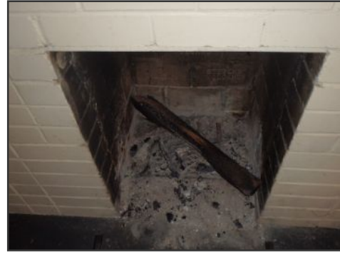
fireplace at bedroom on front
