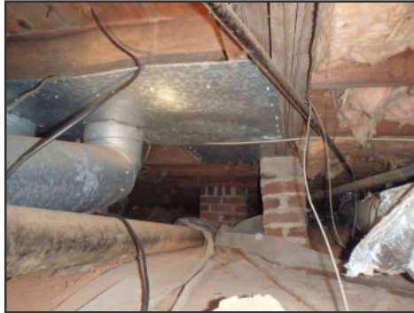
general image of crawl space
