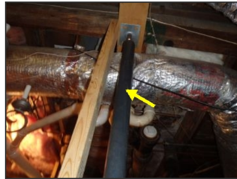
screw jack should be replaced with properly rated post
