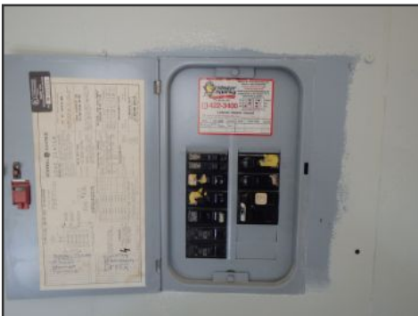
panelboard on right--GE brand
