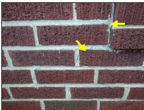
hairline crack at side B
