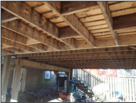
underside of deck
