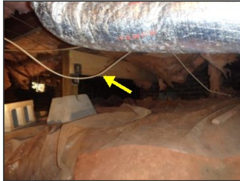
auxiliary beam--posts shifting
