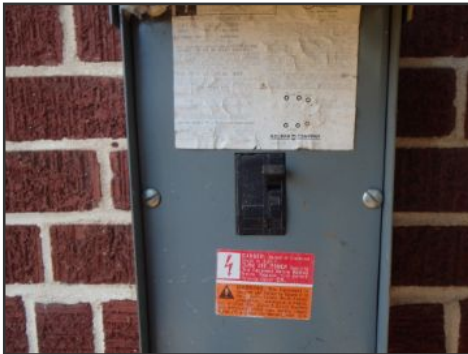
main disconnect B
