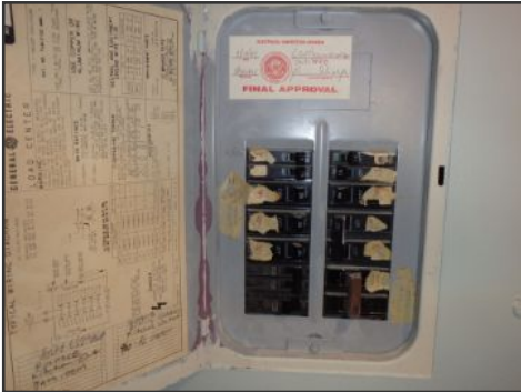
panelboard on left--GE brand
