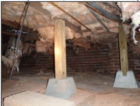
general image of crawl space
