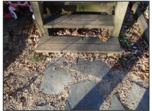
missing concrete landing
