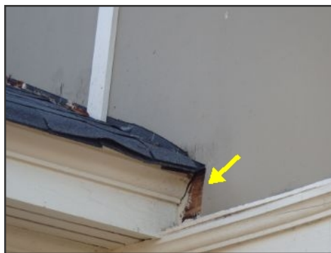
minor wood damage and missing flashing/trim
