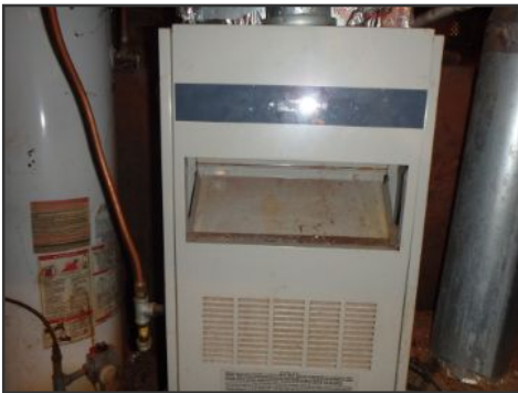
ICP brand furnace--100,000 BTU--25 yrs old
