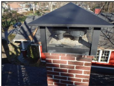
general image of chimney on side B
