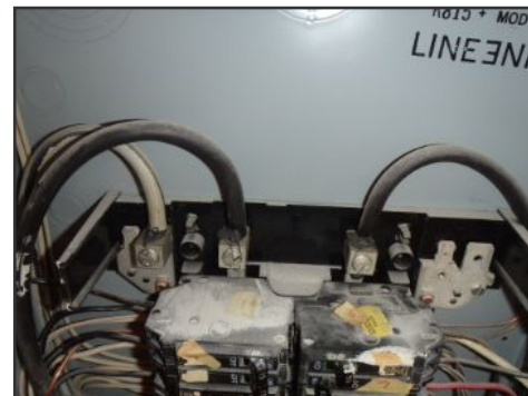
service entrance wiring--right side
