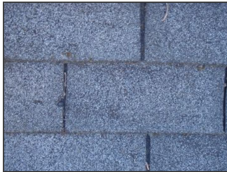
close up of roofing material
