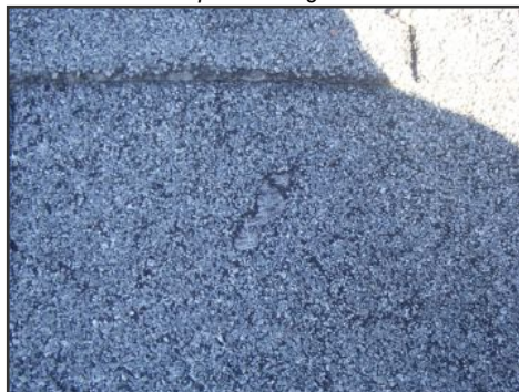
example damaged area
