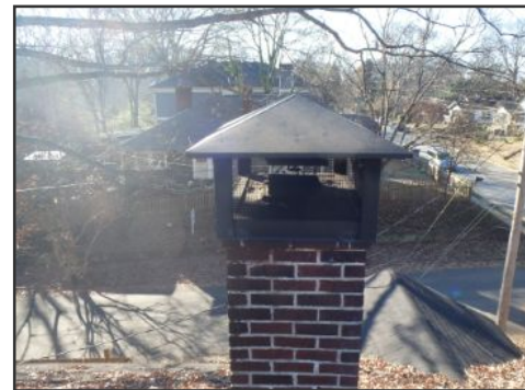
general image of chimney on side D
