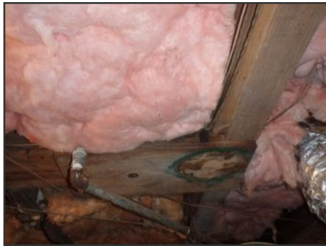
missing support under beam--center of crawl space
