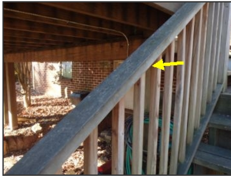
missing grippable handrail
