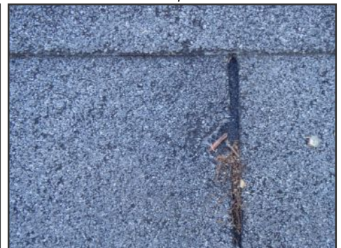
example damaged area
