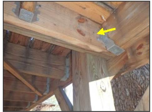
beam/ledger not bolted to post--example
