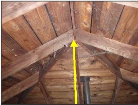
recommend adding strut under ridge rafter tails
