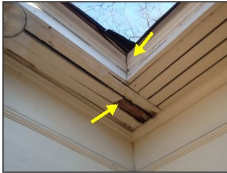
minor wood deterioration at side A
