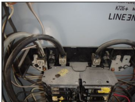
service entrance wiring--right side
