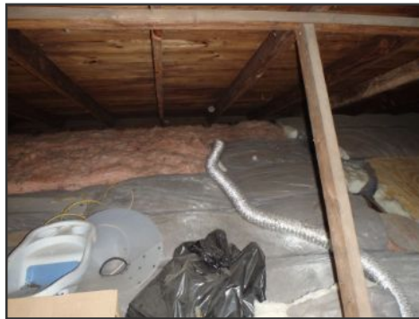
vent does not terminate to exterior
