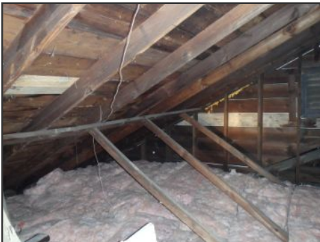
general image of attic framing
