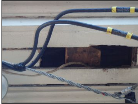
open soffit at side D
