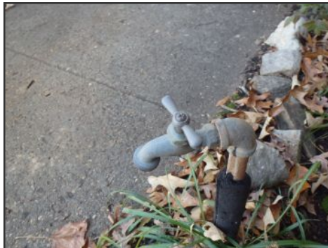
water hose faucet at side A
