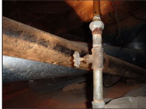
main water valve
