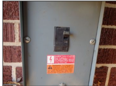
main disconnect B
