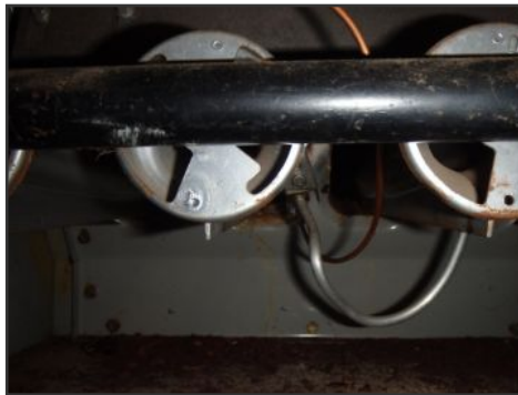
rusted condition of heat exchanger
