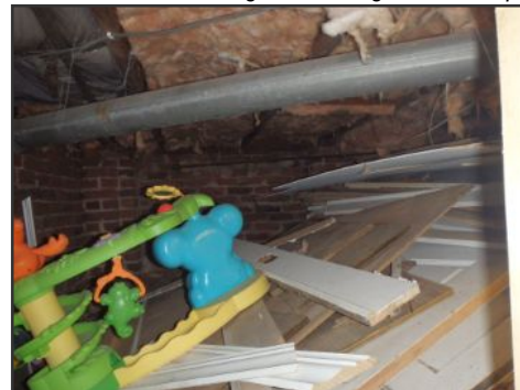
general image of crawl space
