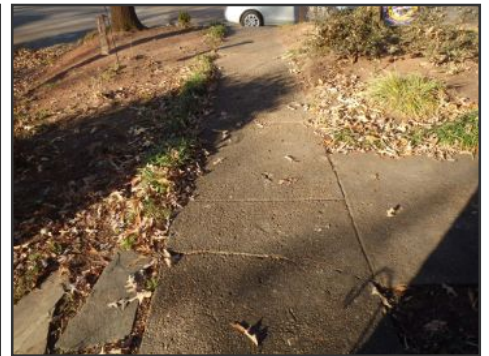
walkway at front
