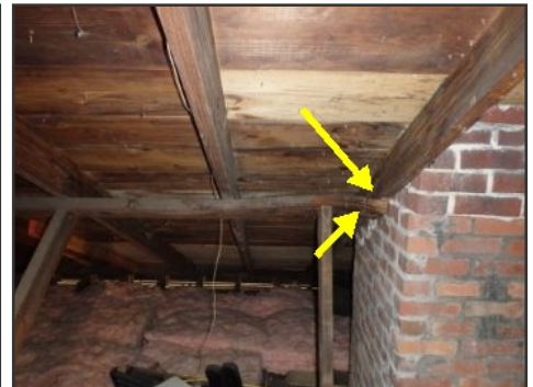
damaged purlin and rafter on side D
