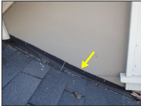
improper vertical wall flashing
