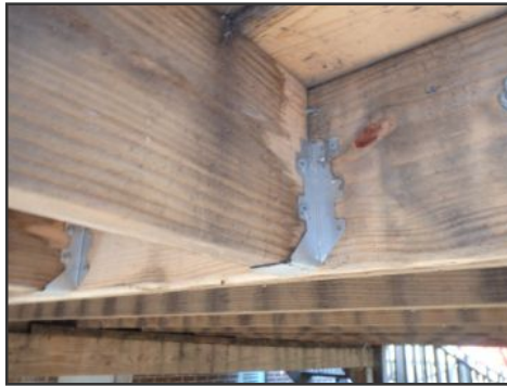
joist hangers undersized and improperly connected with screws
