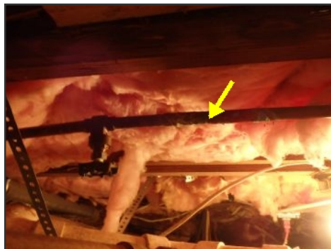
leak at pipe under bathroom
