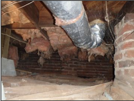
general image of crawl space
