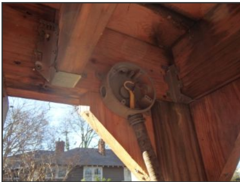
abandoned circuits should be removed
