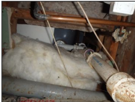
gap under bathroom
