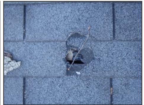
hole at porch
