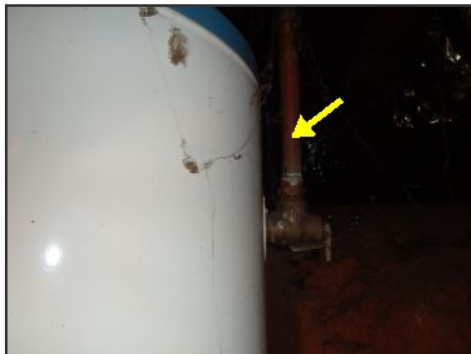
TPR valve discharge tube is improperly installed
