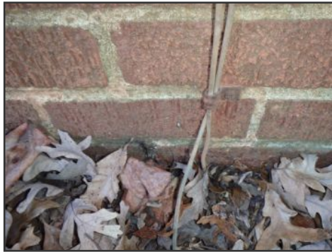
grounding connections
