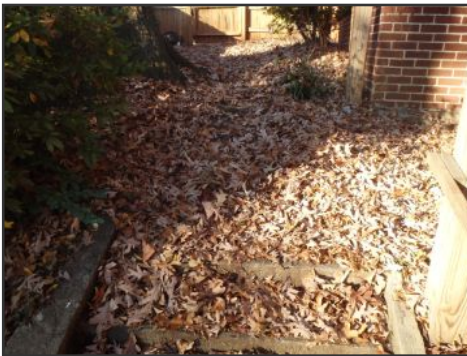
walkway and steps at side D
