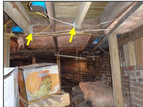
joist hangers improperly installed with screws
