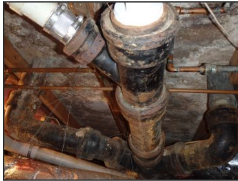
general image of cast iron drain pipes
