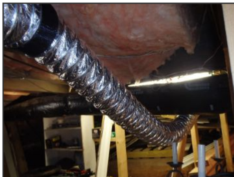
improper dryer duct material
