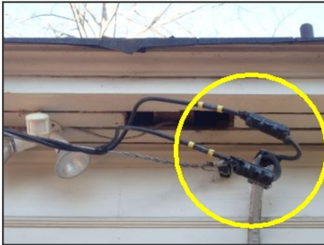
electrical service drop
