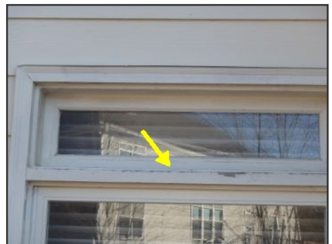
example flaking paint
