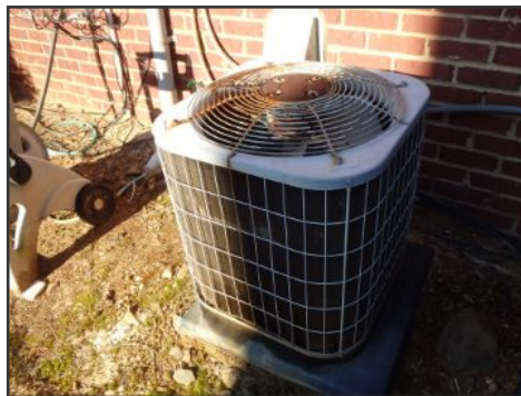
Carrier brand condenser--3.0 tons
