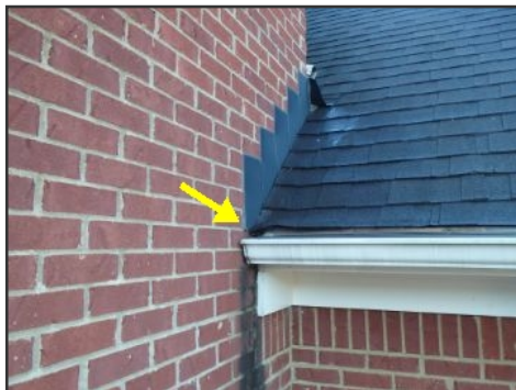
missing kickout flashing
