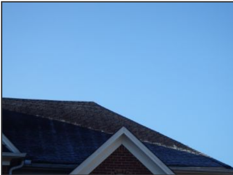
general image of roof covering--side A
