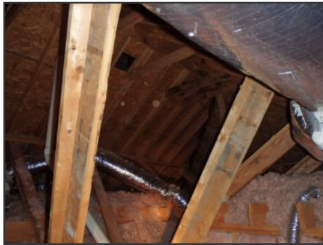
general image of roof framing
