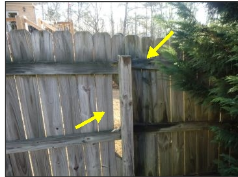
example damaged fence area
