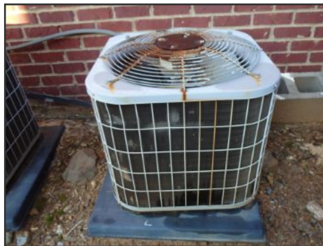
Carrier brand condenser--2.5 tons
