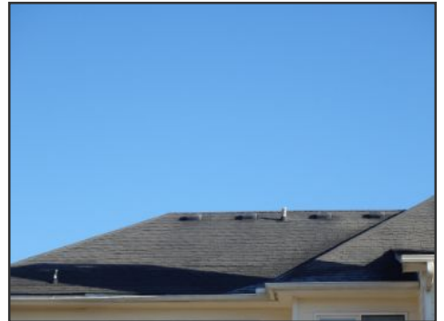
general image of roof covering--side C
