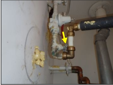
main water valve
