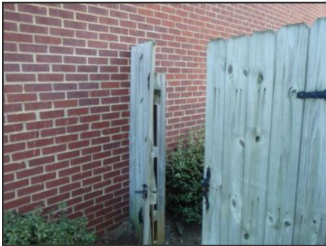
misaligned fence gate
