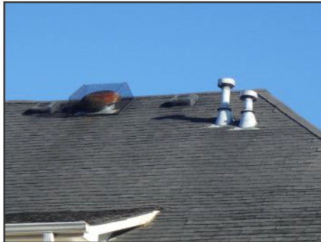
general image of roof covering--side C
