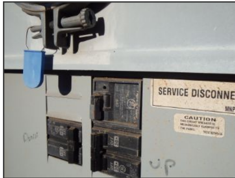
main disconnect--200 Amp
