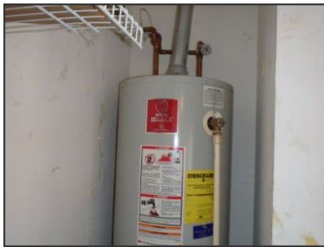
State Select brand water heater--50 gallons
