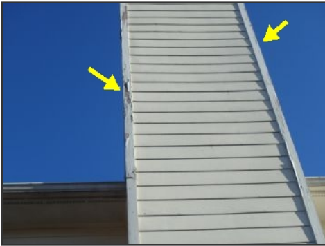
example flaking paint
