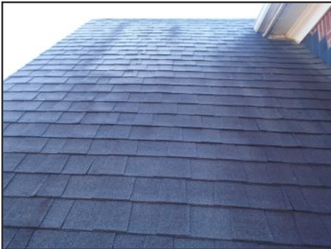
general image of roof covering--side A
