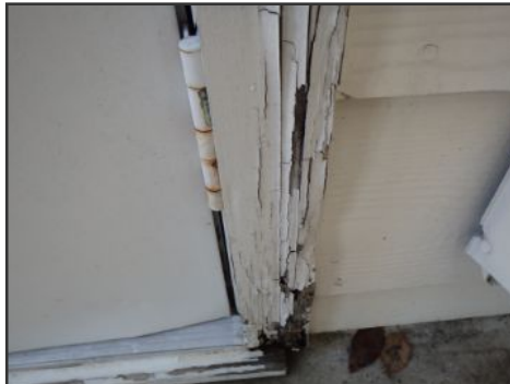
example deteriorated trim--side C
