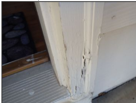
example damaged trim--side C at door
