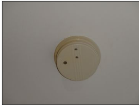
example smoke detector
