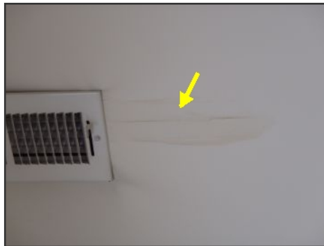
moisture stain--half bathroom
