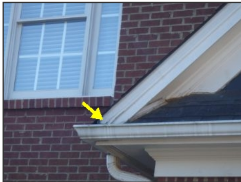
minor fascia deterioration
