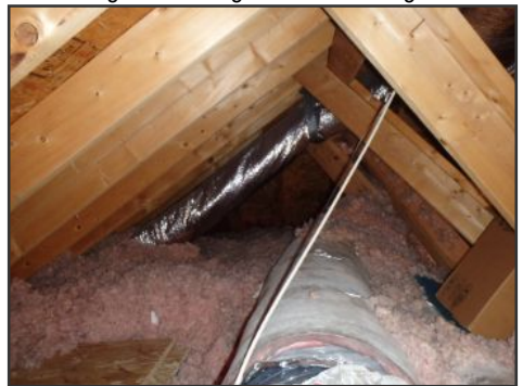
general image of roof framing
