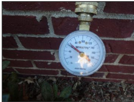
water pressure test
