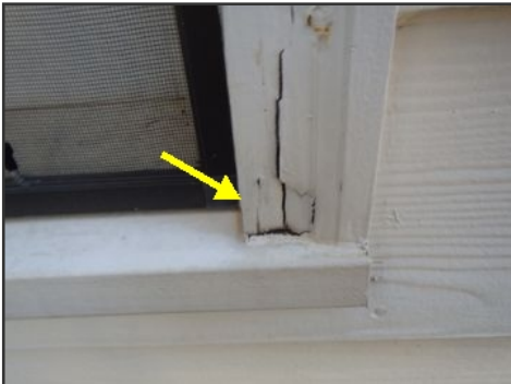
example deteriorated trim--side C
