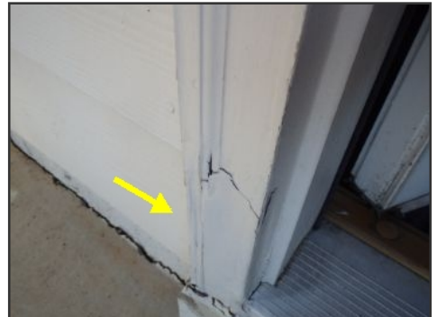
example damaged trim--side C at door
