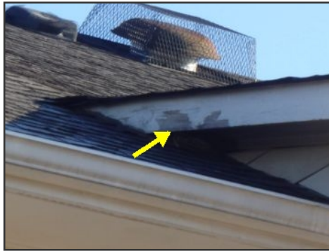
example flaking paint
