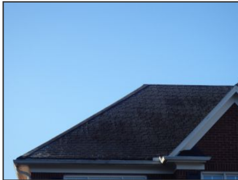
general image of roof covering--side A
