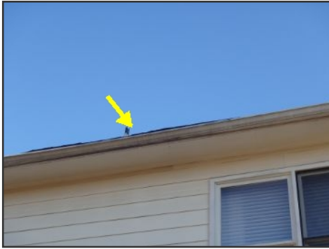
gutter is detaching at side C
