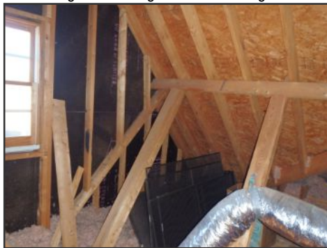
general image of roof framing
