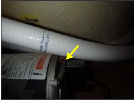
no bonding connection
