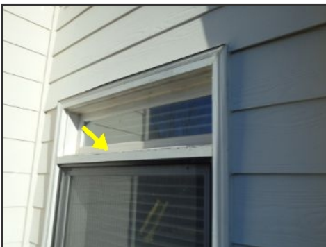
example flaking paint
