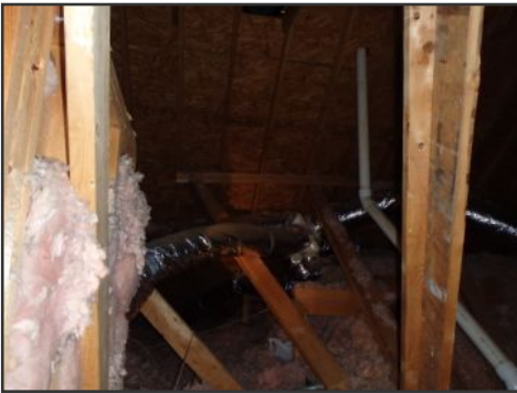
general image of roof framing
