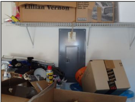
panelboard--located at garage--obstructed from inspection
