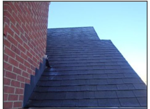
general image of roof covering--side A
