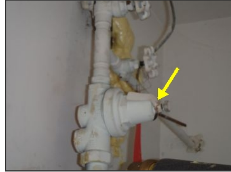
water pressure control valve
