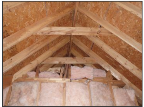
general image of roof framing
