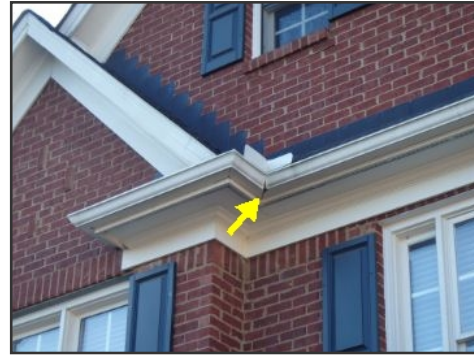
leaking gutter joint example
