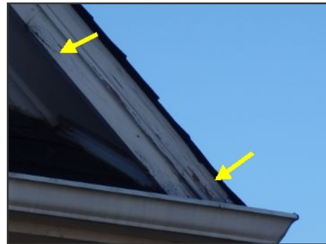
minor fascia deterioration
