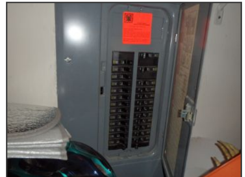
distribution panelboard--Square D
