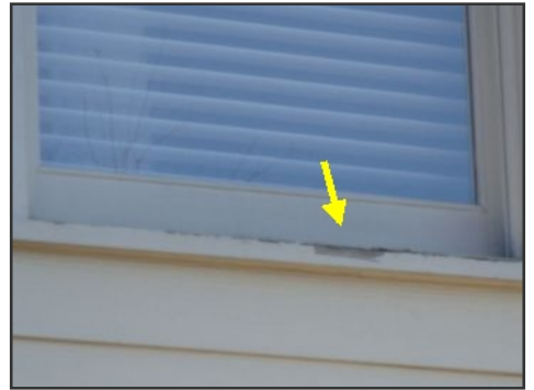
example flaking paint
