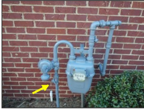
main gas valve
