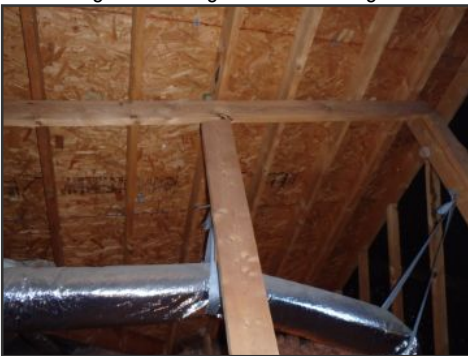
general image of roof framing
