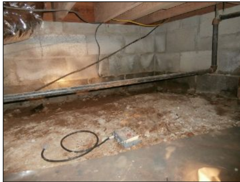
underfloor crawl space--general image
