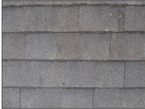
general image of roof covering
