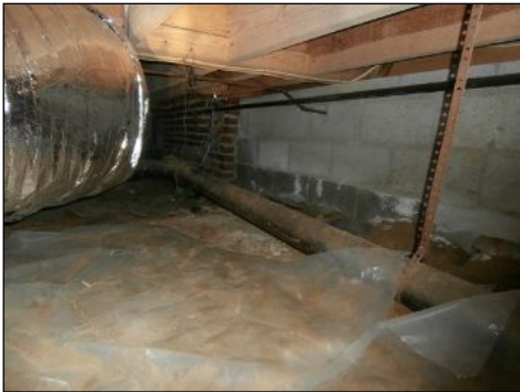
underfloor crawl space--general image
