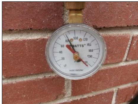
water pressure test
