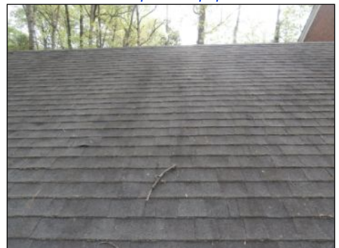
general image of roof covering
