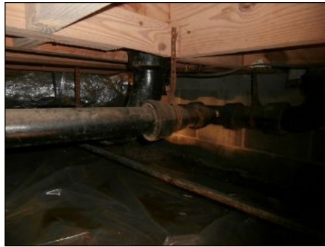
example drain pipes
