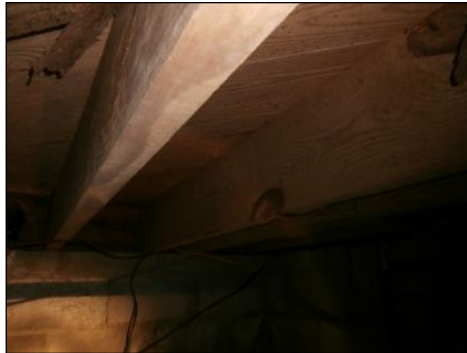
general image of floor system
