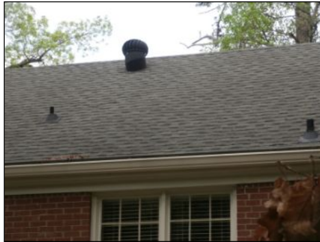
general image of roof covering
