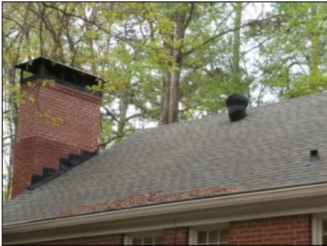
general image of roof covering
