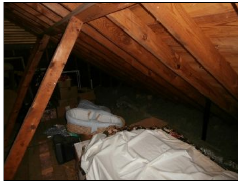
general image of attic
