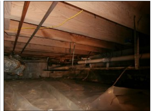
underfloor crawl space--general image
