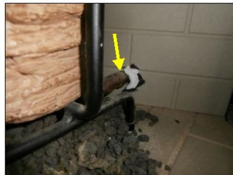
*proper sealant should be installed*
